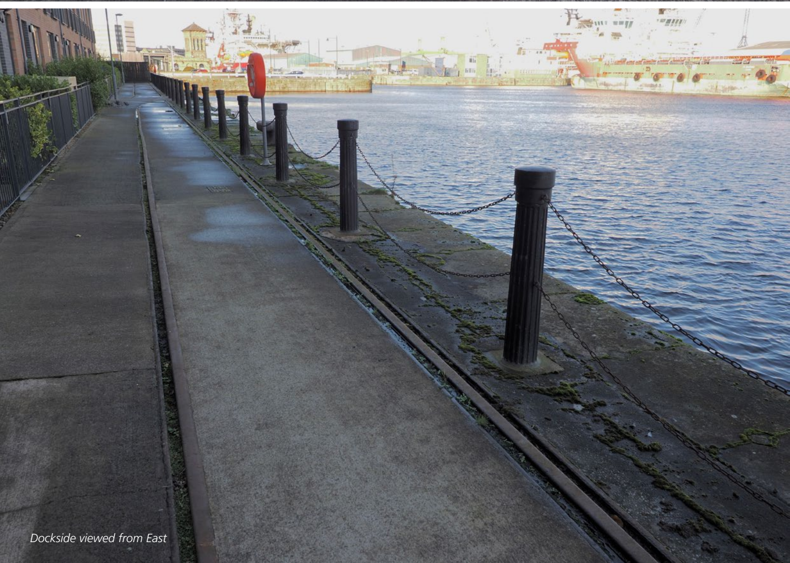
Existing Bollards and Chain fence
