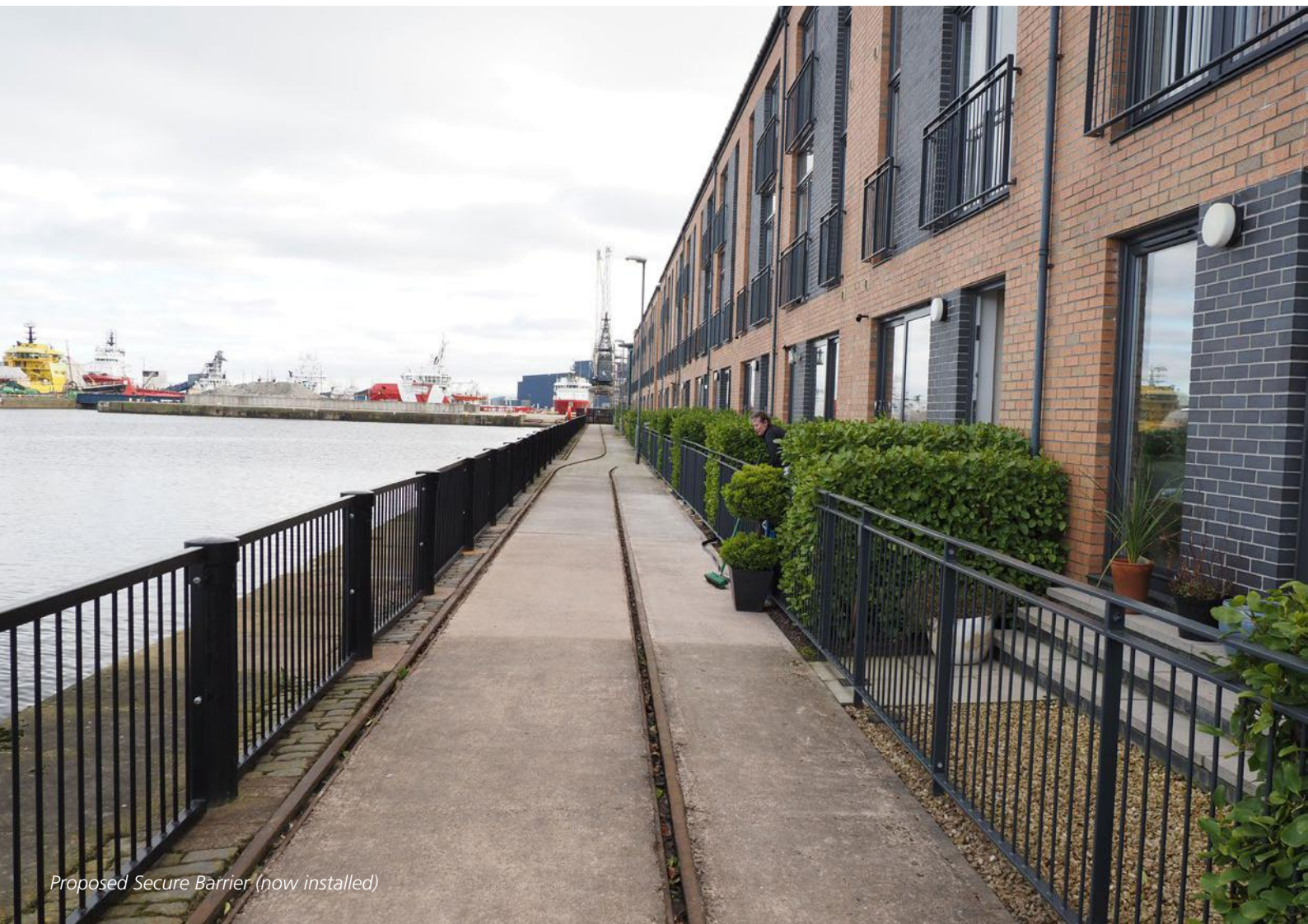
Dockside prior to installation of Secure Barrier
